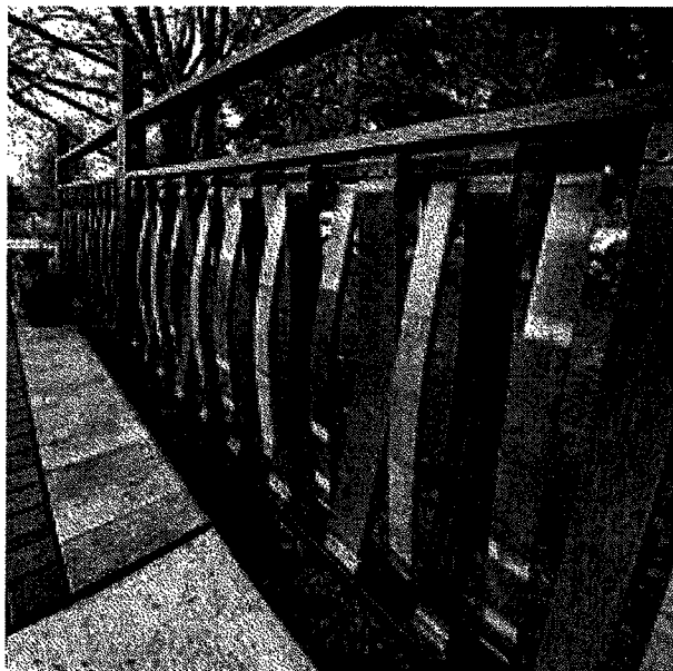
Image 6: Example decorative barrel stave fence (max. overall height of six feet) at Location Key 'D'
